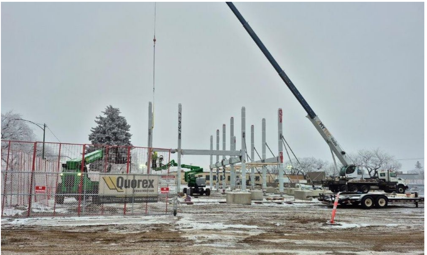
Image 2: Installation of columns and beams
