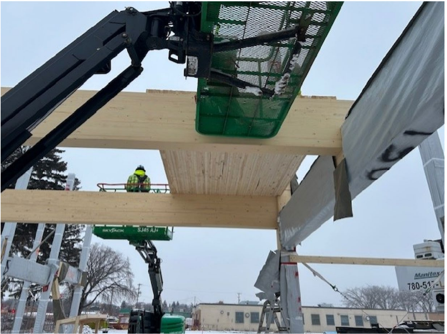
Image 3: Installation of reclaimed NLT
